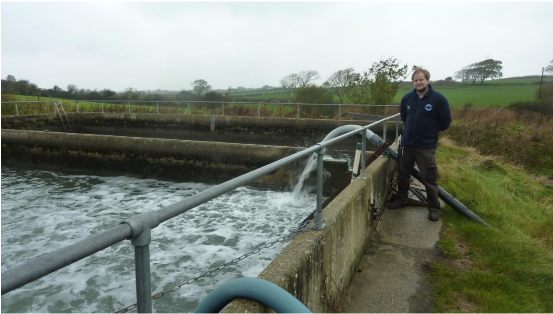
This is senior aquarist Matt Davidson with the inlet pipe that is pumping seawater from the Menai into the large settling tank.
