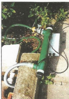
The author's UV steriliser disconnected ready for installing a new lamp — note the outlet pipe is larger than the inlet, another tip for good water flow through the unit.
